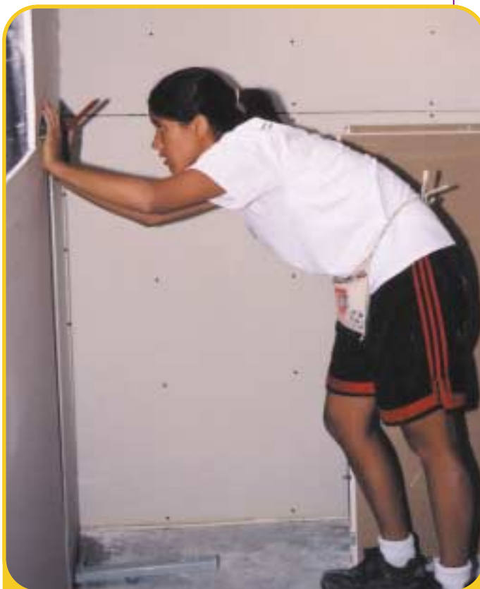
Natasha takes measurements for the next sheet of drywall.
