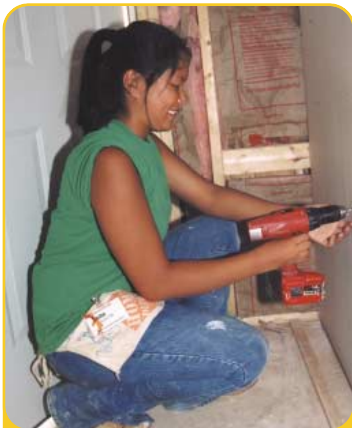
Sasha secures the drywall in the new living room.
